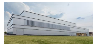
Neubau Physical Fitness Center, Katterbach
