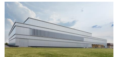
Neubau Physical Fitness Center, Katterbach
