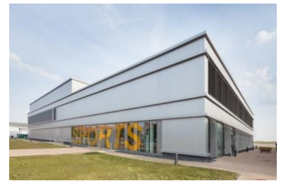
Physical Fitness Center, Katterbach
