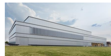
Neubau Physical Fitness Center, Katterbach
